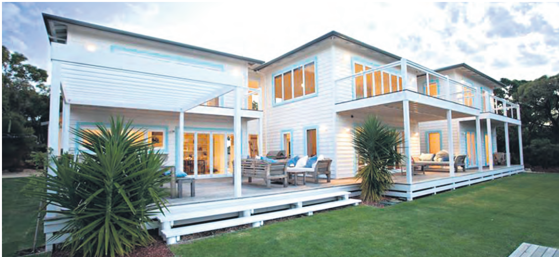
Cedar weatherboard cladding was used on the exterior, with Alaskan yellow cedar used on the home's patio.
